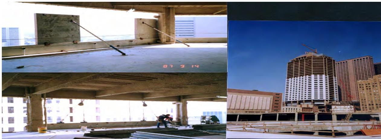
FIGURE 3.2 Example of a prefabricated exterior paneling system. SOURCE: Thomas (2008).
